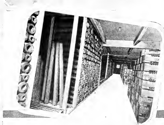
BUILT-UP COLUMN WAREHOUSE
